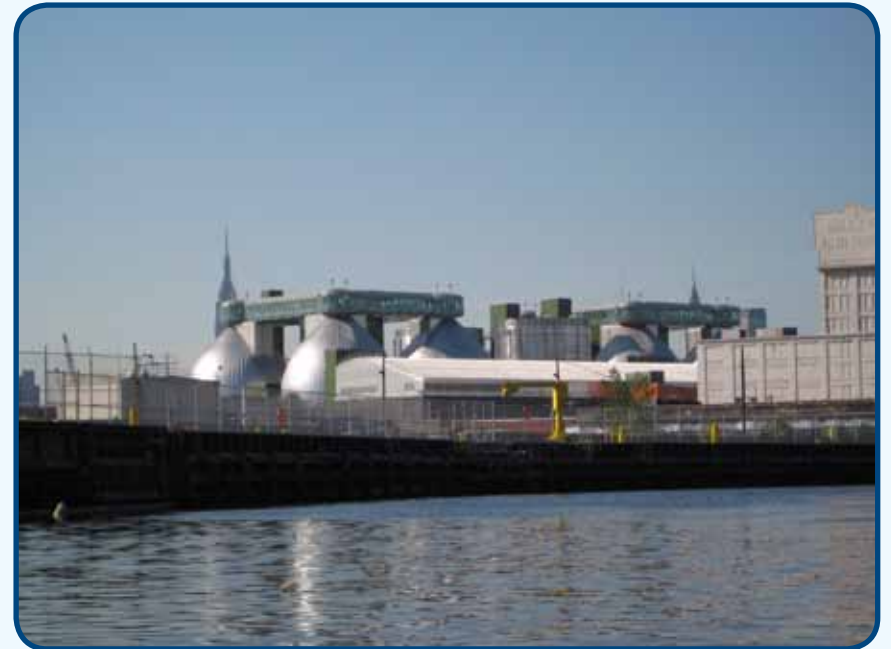
Newtown Creek Sewage Treatment Plant, Brooklyn.
