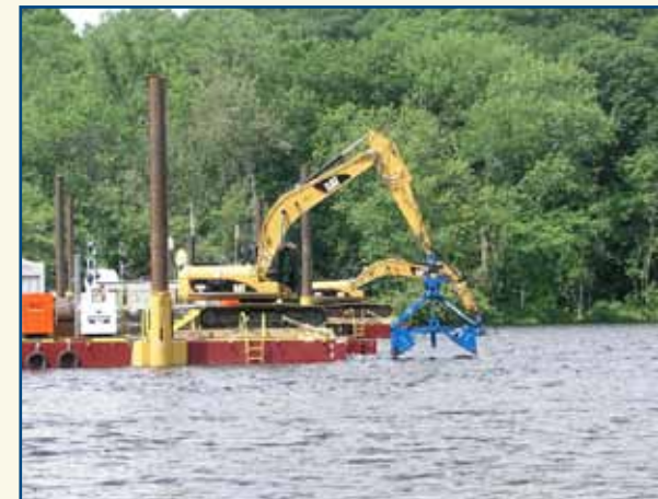
Removing contaminated soil with dredgers.
